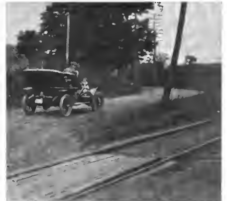
CROSSING IN LIMITS OF BRIARCLIFF.
